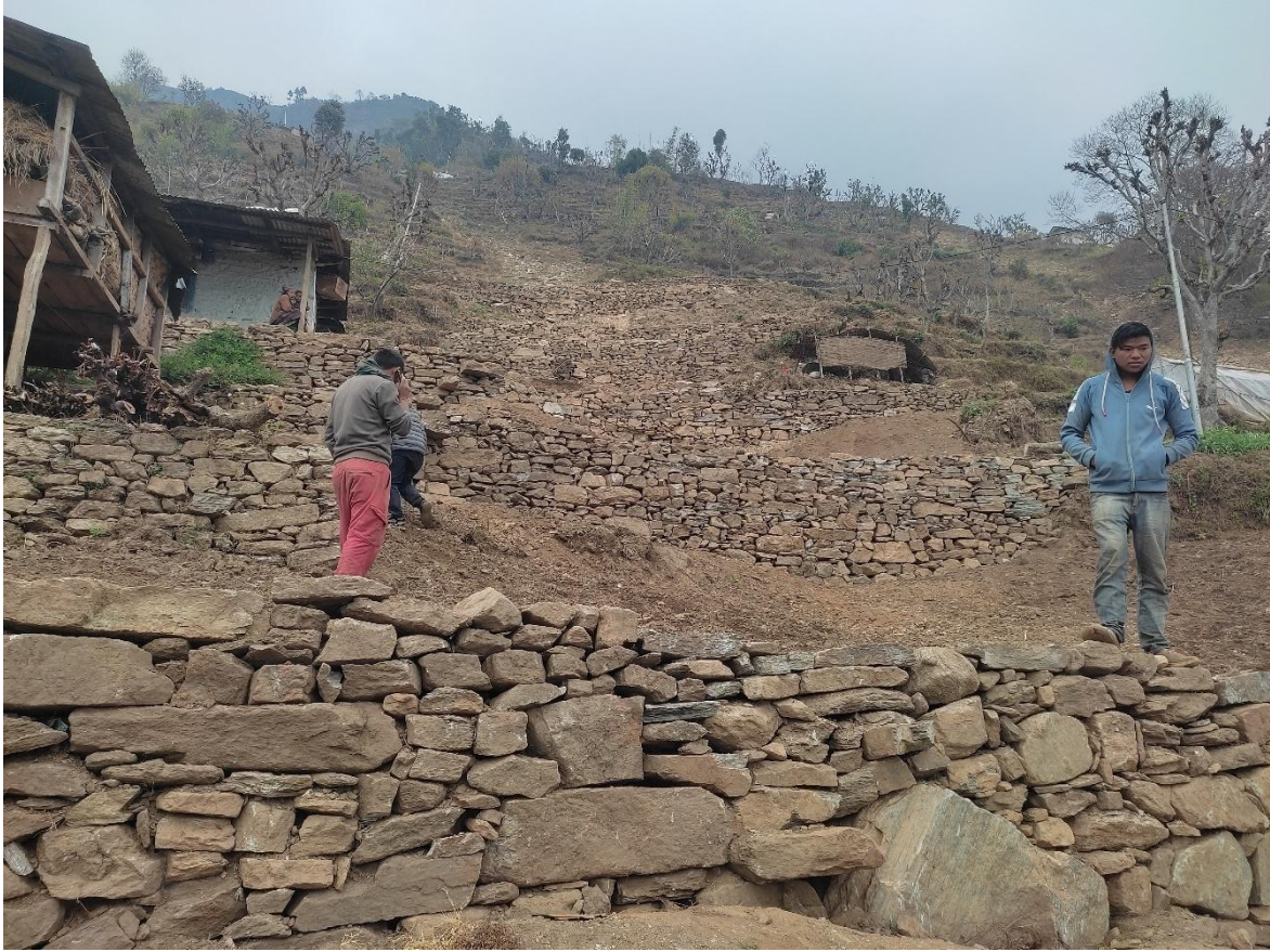
Figure 15: Dry stone stacked wall constructed by locals to intercept debris flow
