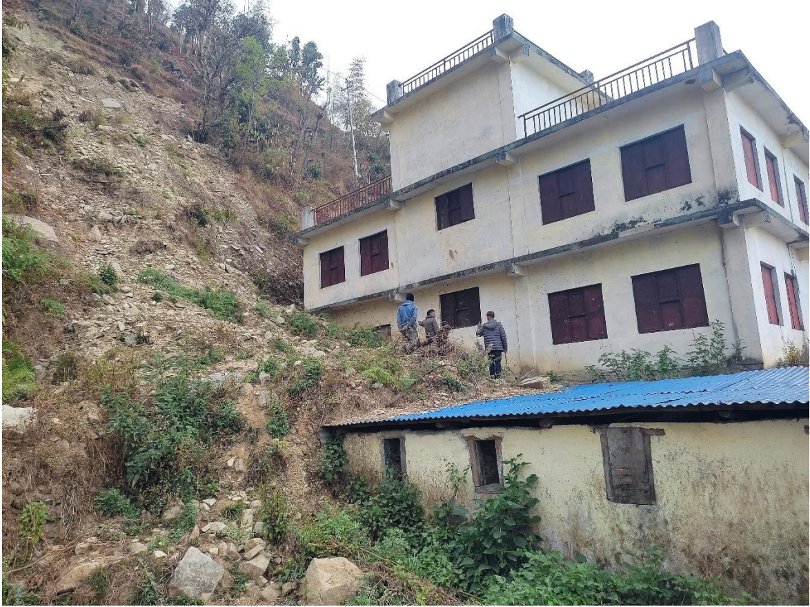
Figure 14: Debris flow deposit to the side of building constructed for school and on roof of toilet
