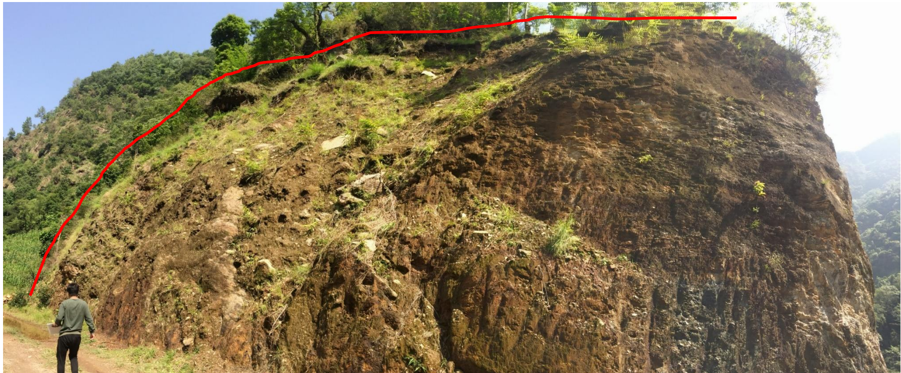
Figure 5: Picture showing Landslide on upslope of road
