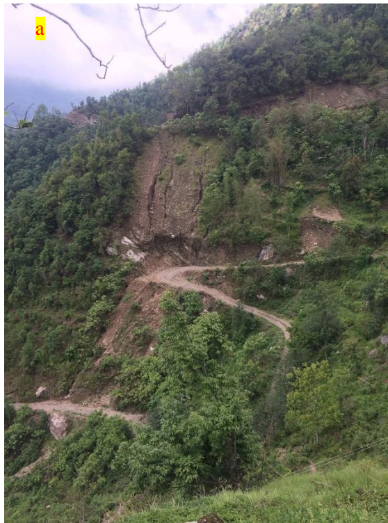
Figure 18: Picture showing (a) shallow landslide due to road cut and (b) presence of rock outcrop in top part
