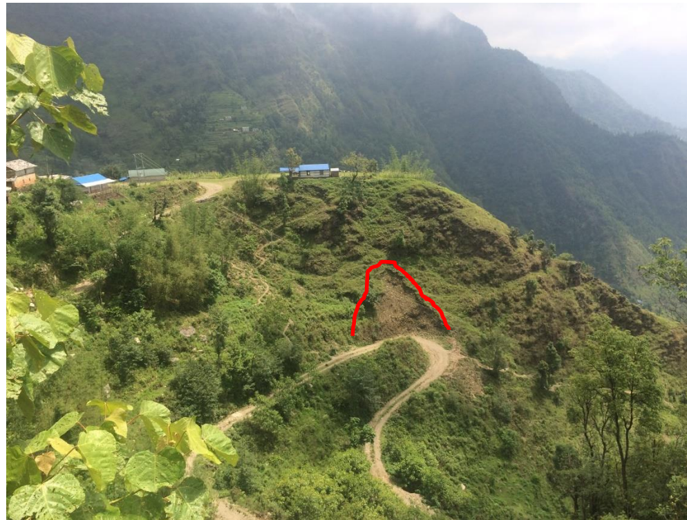
Figure 17: Picture showing shallow landslide due to road cuts. There is health post on top part
