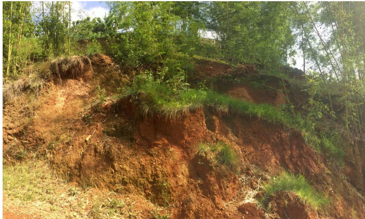
Figure 21: Picture showing landslide with mud fall
