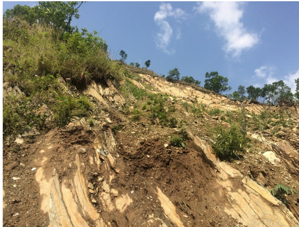
Figure 15: Picture showing landslide with rock exposure
