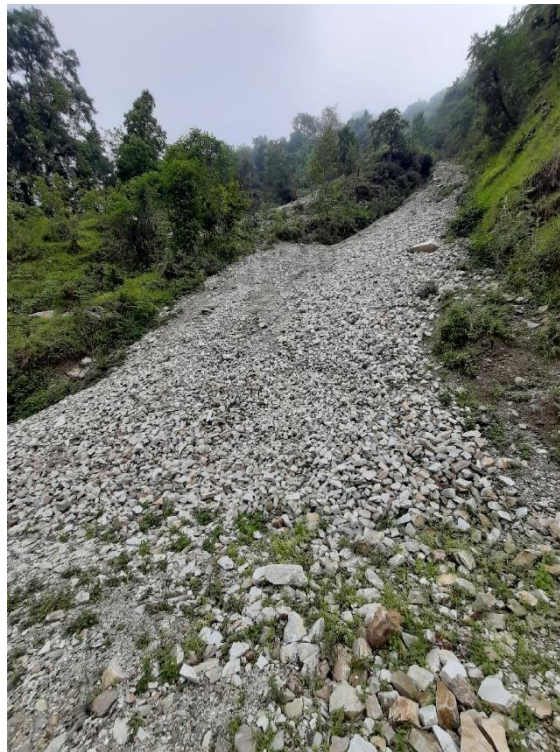
Figure 11: Picture showing debris flow from road cut in Saimal
